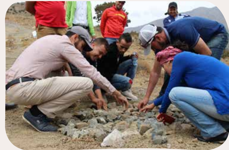
Figure 5.1. Building a one rock dam
